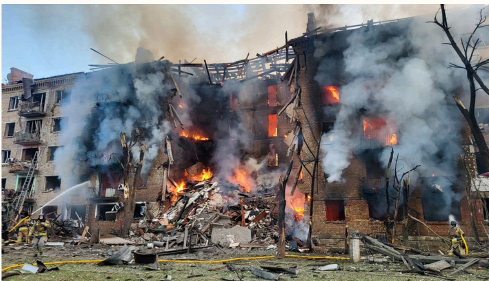
Firefighters extinguish a fire in an apartment building partly destroyed by a Russian strike in Kyiv. [Global Images Ukraine] Source: The Guardian
